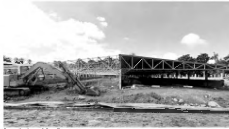
Installation of Roofing
