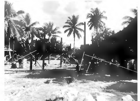
I-Beam Foundation Setting
