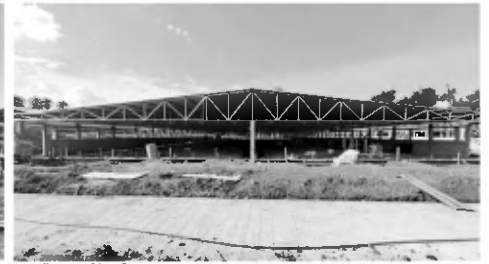
Installation of Roofing
