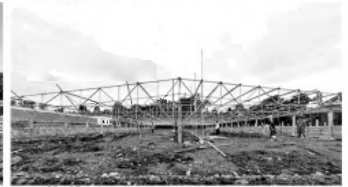
Setting of Roof Foundation
