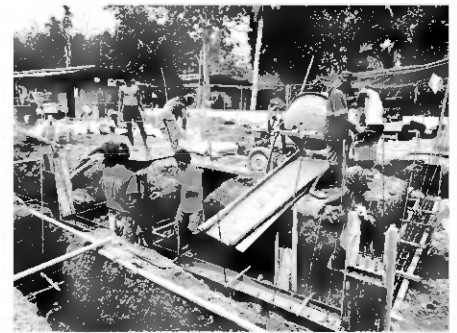
Foundation Concreting
