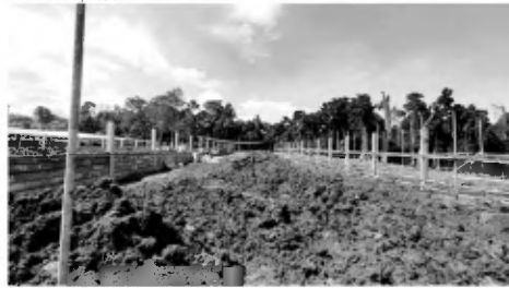
Erection of Foundation
